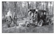
Back in 1950 new technology and more efficient means were developed to help combat wildfires. TFS crew leaders Surcey Peoples and Bob Williams demonstrate how to use a Jeep equipped with a fire plow. They also used a drip torch to set a backfire and remove any flammable fuel near the plowed fire lane.
