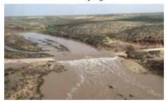
The Pecos River above the Red Bluff Reservoir. Wet areas show how much higher the water had been in the hours prior. It is still flowing a lot of water and has washed out this oil field road. The black poly line you see on the left across the road and on the right in the river bed is an oil field line that used to stretch across the river and as you can see it was separated from the force of the water. Road damage is visible at the current water's edge on both the left and right sides.
