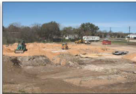
March 2013 - Construction Site
